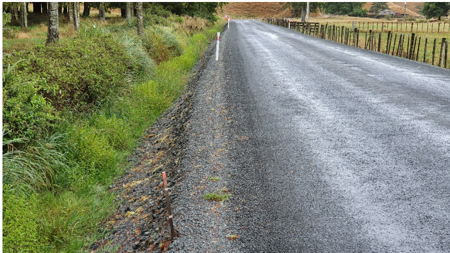
Figure 6 Taharoa Rd Rehabilitation site
